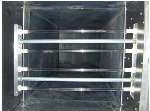
Figure 2-2. Device installed inside the test rig. There are 4 lamps and 2 support rods.
