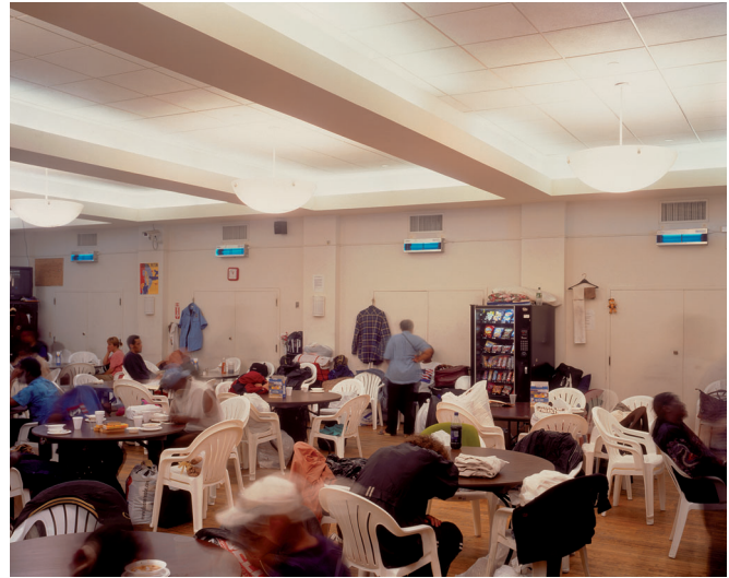
Figure 6. Wall-mounted UVGI fixture used in the St. Agnes Shelter for the Homeless (Atlantic Ultraviolet Corporation Hygeaire™ model LIND24-EVO)
