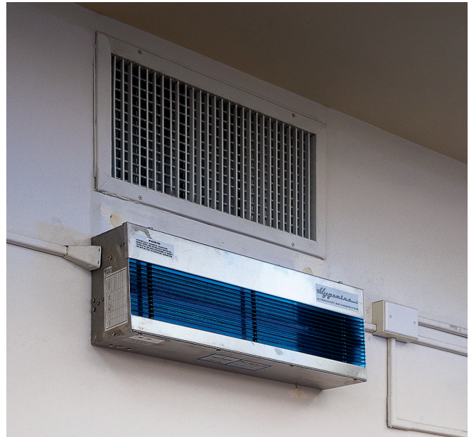
Figure 6. Wall-mounted UVGI fixture used in the St. Agnes Shelter for the Homeless (Atlantic Ultraviolet Corporation Hygeaire™ model LIND24-EVO)
